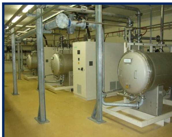
Ozone generator building
