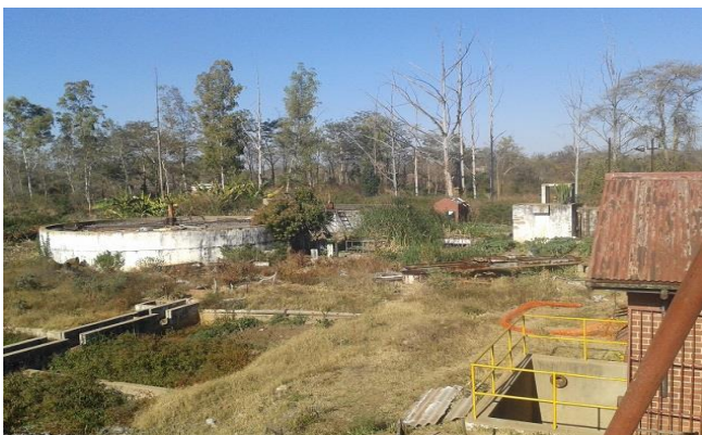
Figure 1 Current State of the Redcliff Wastewater Treatment Works.
