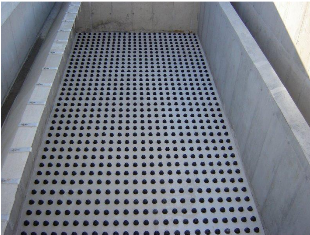
Floor cast and stems and domes installed, pre media installation.
