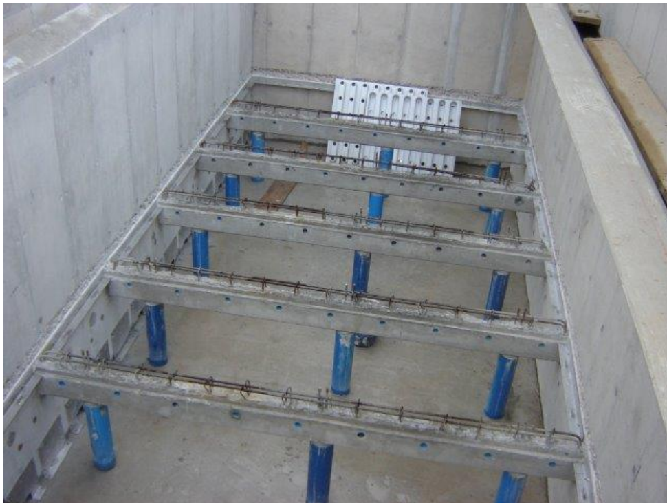
Support columns and beams.
