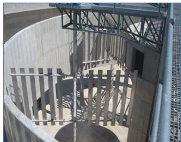
Flocculator paddles after installation
