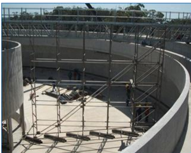
Clarifier scraper mechanism during installation
