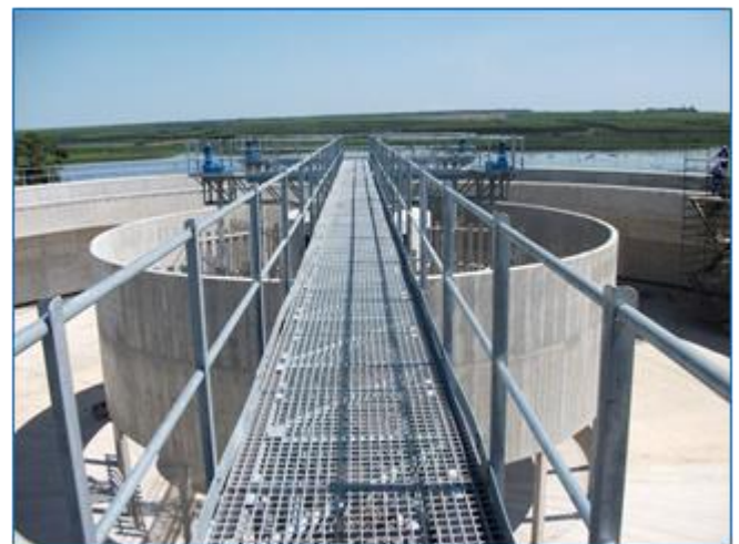
48m diameter clariflocculator after installation
