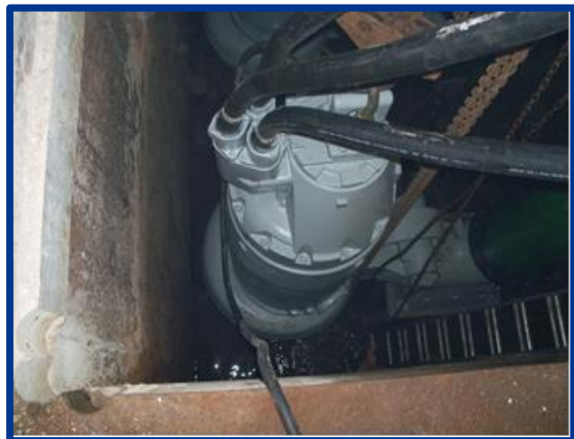
Pump in the process of being installed into the sump.
