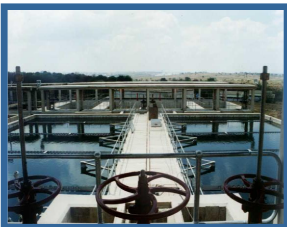
FLAT BOTTOM CLARIFIERS IN OPERATION
