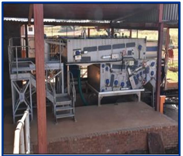
1 off dewatering system (complete with filter belt press, polyelectrolyte dosing, pumps and compressed air system)
