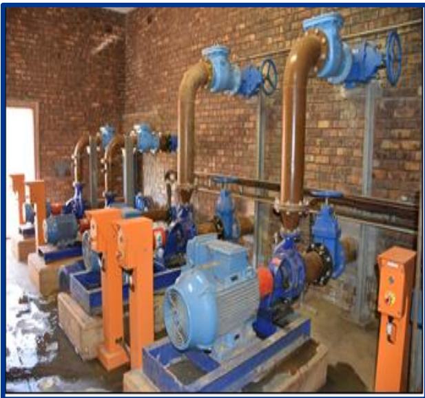
6 off axial flow internal recycle pumps
