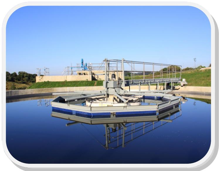
**ROTATING BRIDGE CLARIFIER WITH DOUBLE STILLING WELL**
