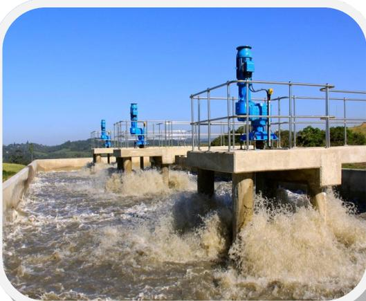
A multi bladed impeller driven by a heavy duty seamless tubular shaft, is suspended in the tank from the vertical output shaft of a generously rated gearbox. The PCI aerator is robustly configured to ensure that the blades radiating from a centre shaft are well supported and shaped to prevent rag accumulation. The drive is selected to deal with axial and radial loads imparted by the suspended aerator using generous service factors to ensure a long service life with reliable operation.
