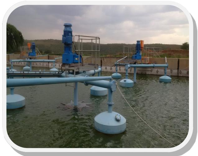
PCI Aerators are available as fixed bridge mounted units or as floating aerators where a tri-float arrangement is used to keep the device at the water level selected for the particular duty. The power of the aerator is selected to suit the requirements of each case and aerator designs are available to suit all motor sizes up to 110 kw.
