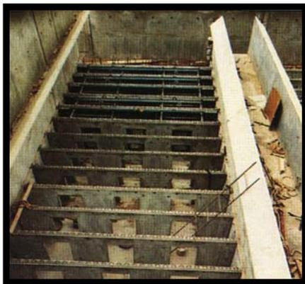
3. Form dwarf walls using either traditional or modern formwork methods or use PCI's optional pre-formed permanent wall formwork
