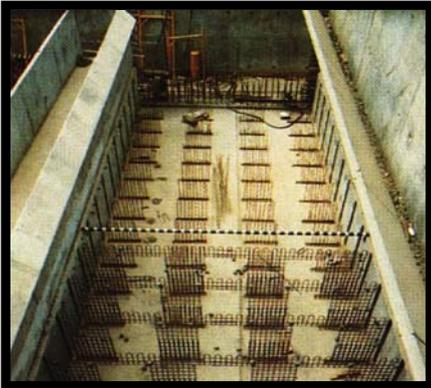
2. Construct filter shell to Engineer's requirements, leaving starter bars in the base for dwarf walls and rebates in the side-walls
