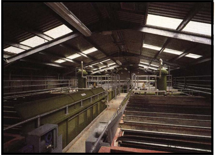
*Twin air absorbers and chain/flight skimmers*
