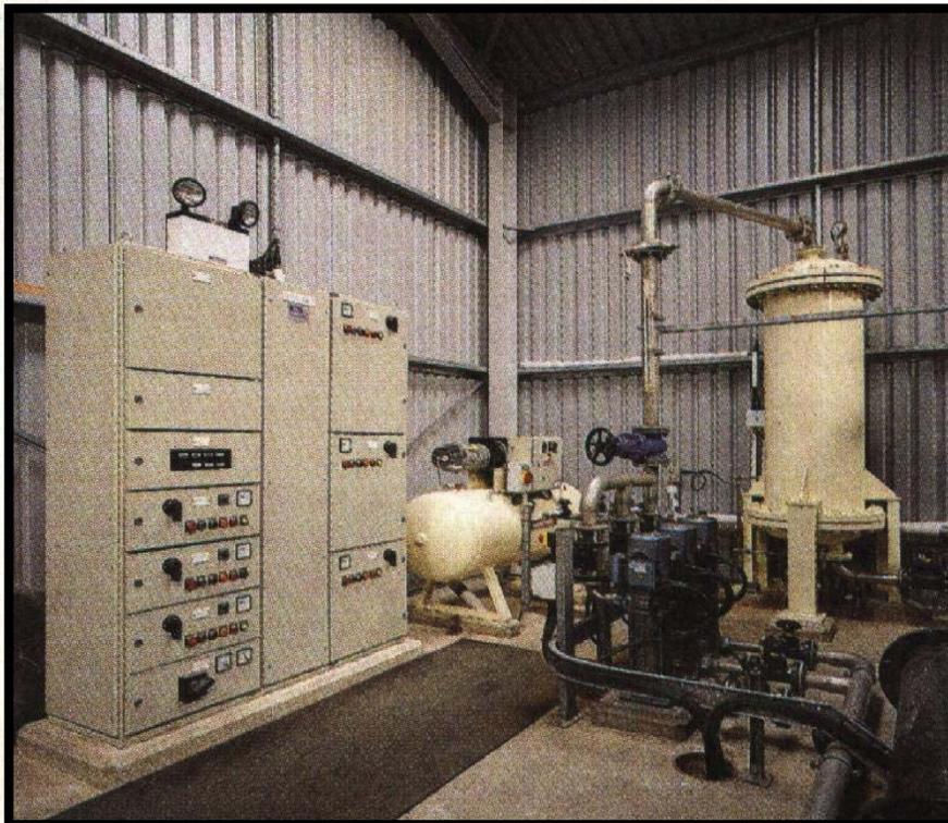
*Water recycle pumps, air compressor and packed absorber vessel.*
