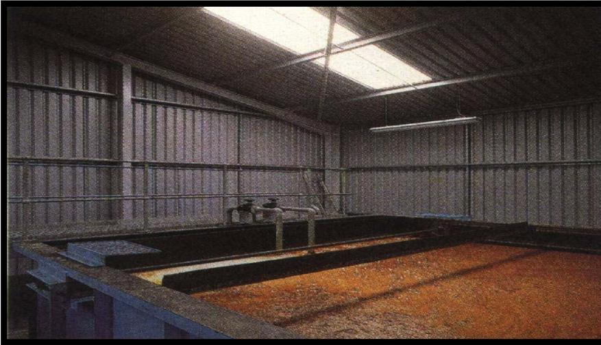
*Air bubbles emerging at the inlet end of a flotation clarifier*
